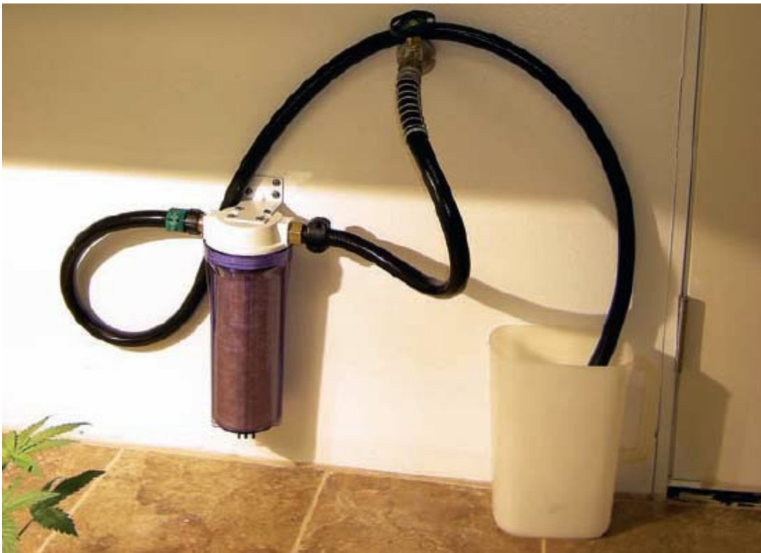
Single carbon filters can work with low PPM water
